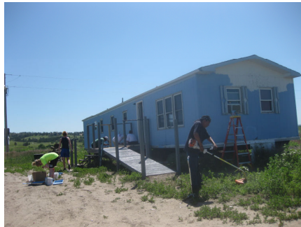
Working on home repairs
